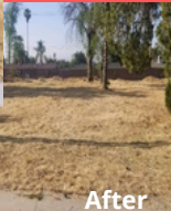
Vacant Lot Clearing on Sunrise Lane
